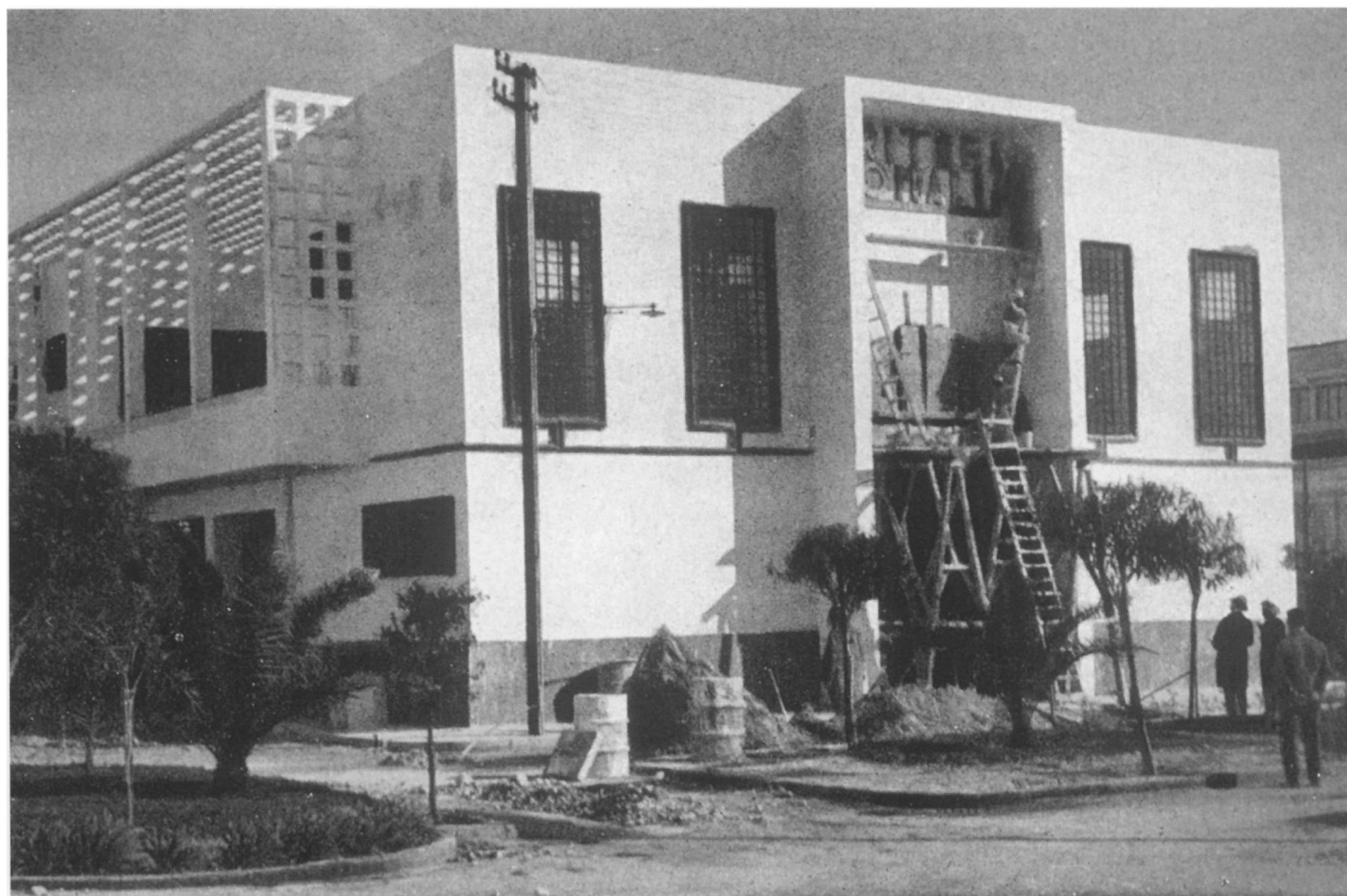
Fig. 12. Sebastiano Larco and Carlo Enrico Rava, pavilion of Eritrea and Somalia, Tripoli Trade Fair, 1934, view. (Photo: from Rassegna di Architettura 6, 7 [July 1934]: 281)
